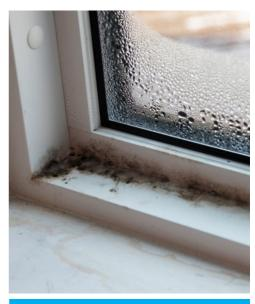
High levels of moisture in one room (such as the kitchen or bathroom) can result in condensation occurring in other parts of the house, especially in cold rooms.
