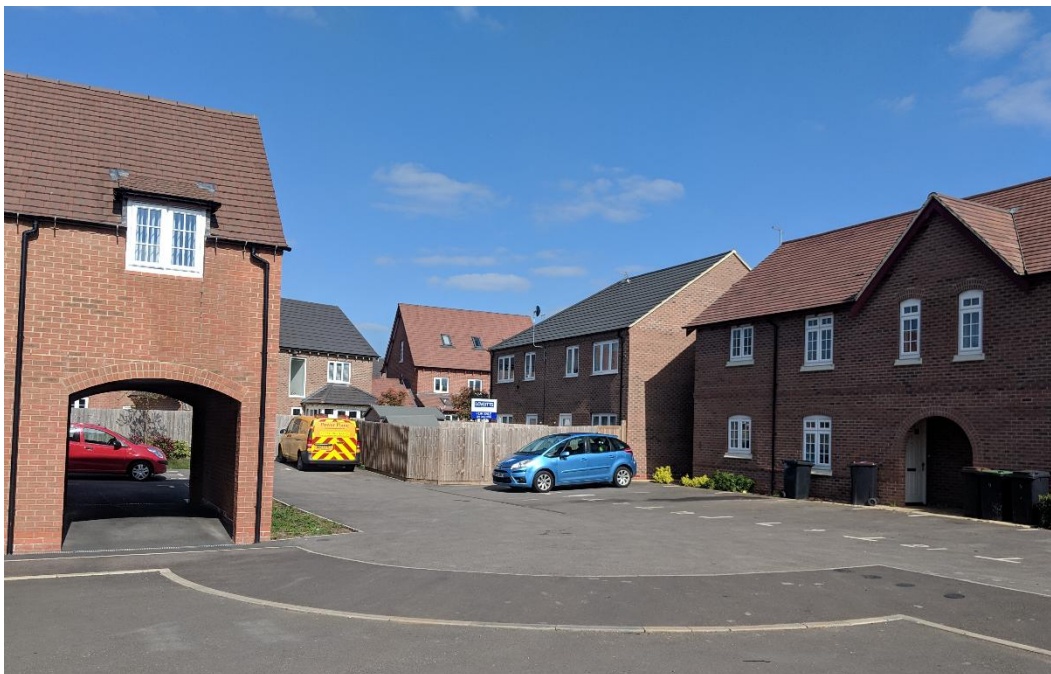
Figure 10: North Nuneaton, flat over parking
