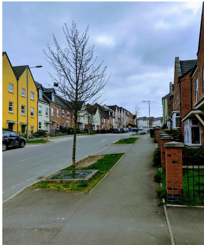
Figure 5: Redevelopment of Camp Hill, Nuneaton demonstrates traditional red brick designs with occasional pastel-coloured buildings, with varying designs providing visual interest.
