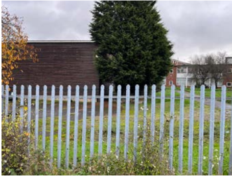
View of disused buildings within the site
