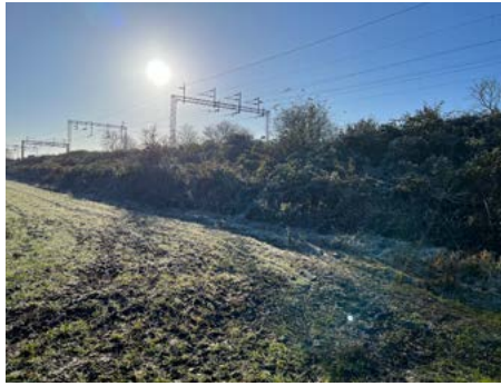
View of railway embankment to west of site
