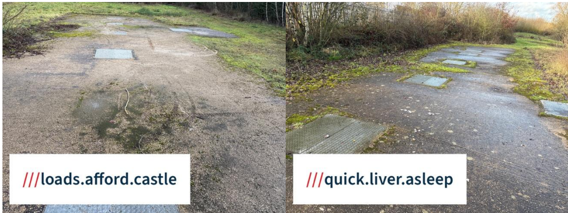
Photos 16 and 17. Severn Trent oil filters
