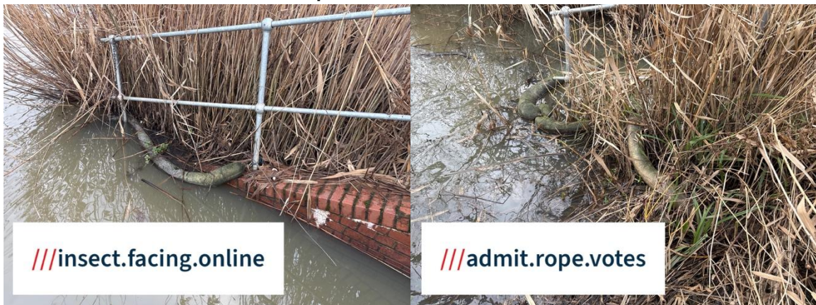
Photos 12 and 13. Spill booms/socks around culverted inlets
