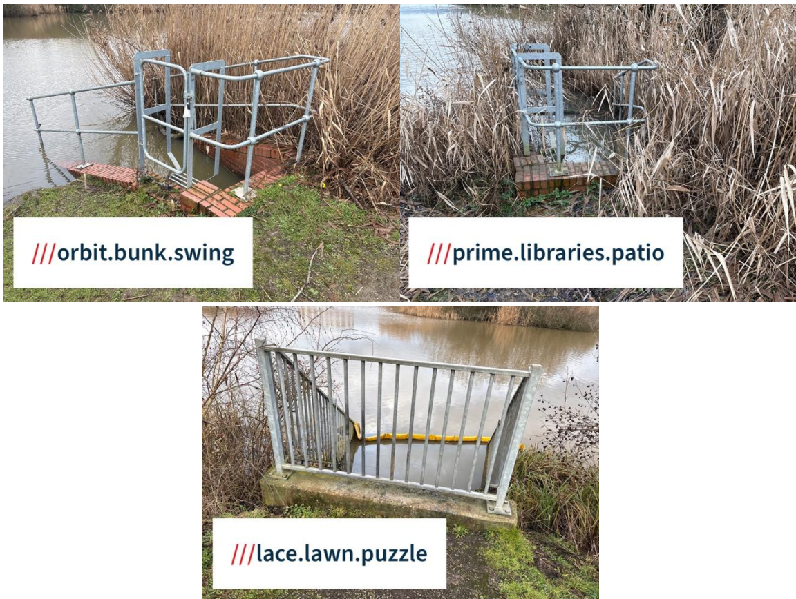
Photos 7 to 9. Culverted inlets
