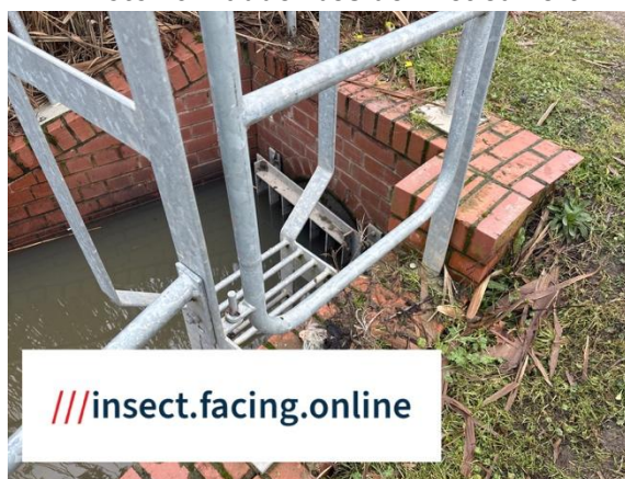
Photo 19. Ladder beside inlet culvert
