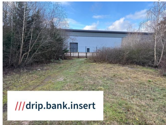
Photo 18. Former access point to oil filters blocked off during recent development
